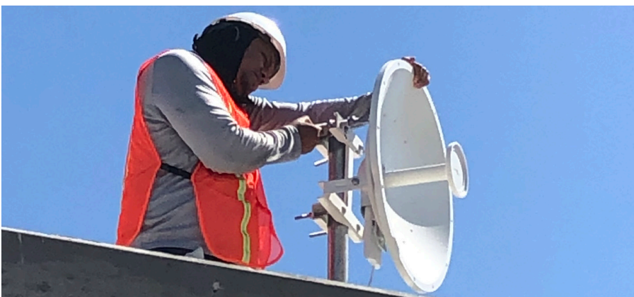
Fixed wireless equipment adjustment
